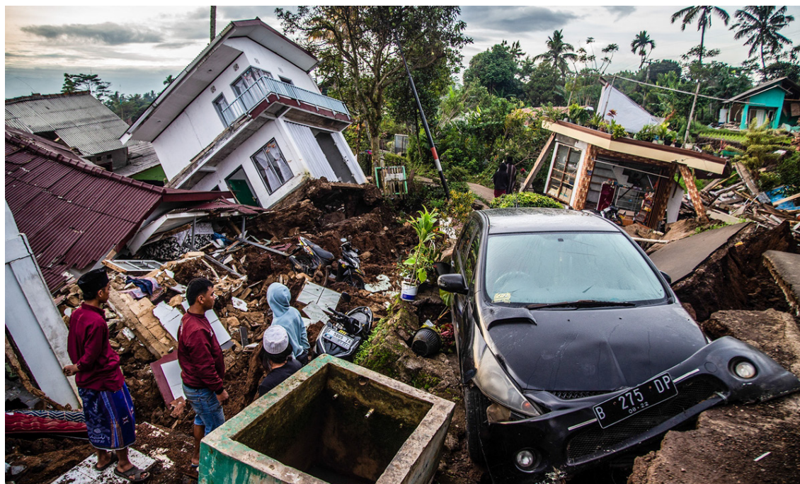
Photo: Earthquake damage in Indonesia, 2022, MPBI
