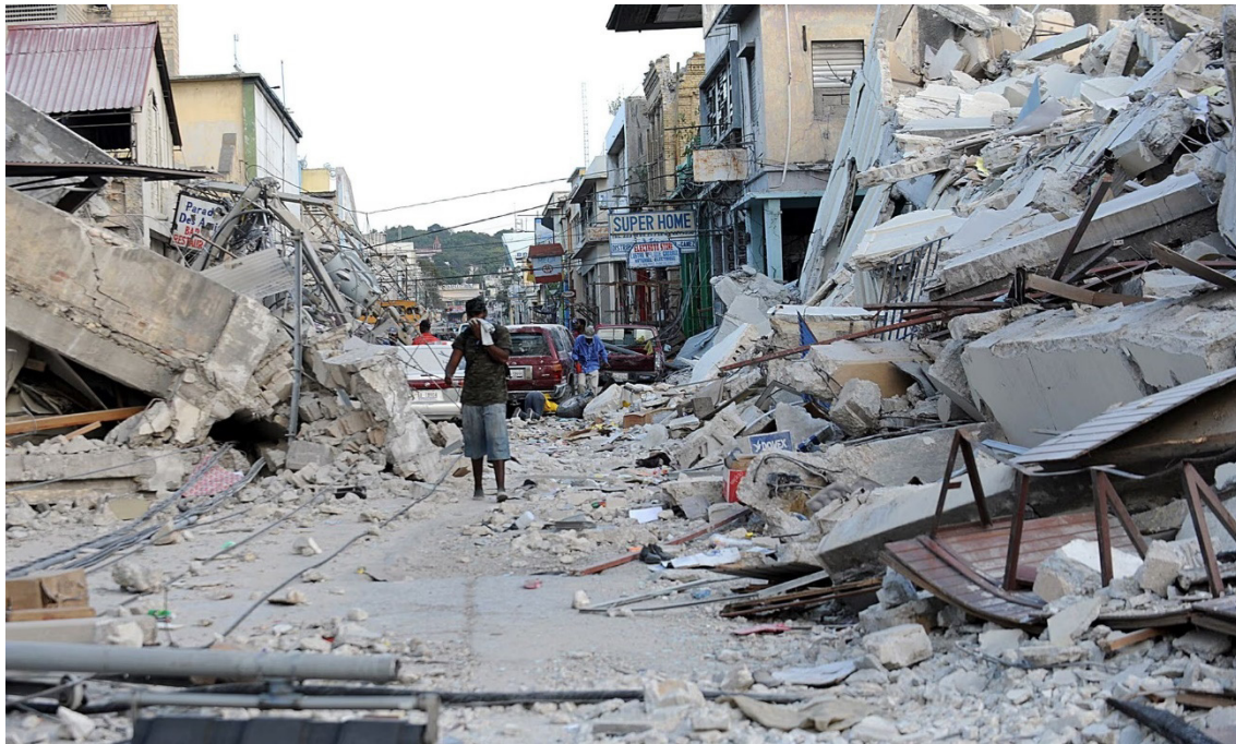
Photo: Earthquake damaged building in Haiti, The Guardian
