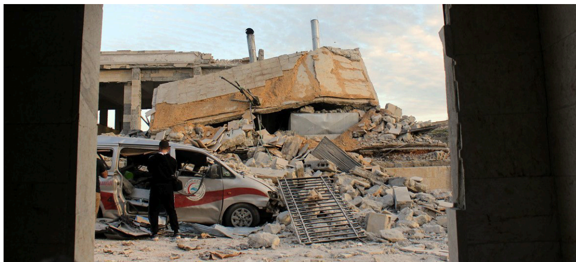
Photo: Damaged health infrastructure in Syria, UN News Agency
